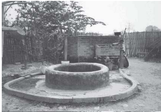
Fig. 8 Private water well
